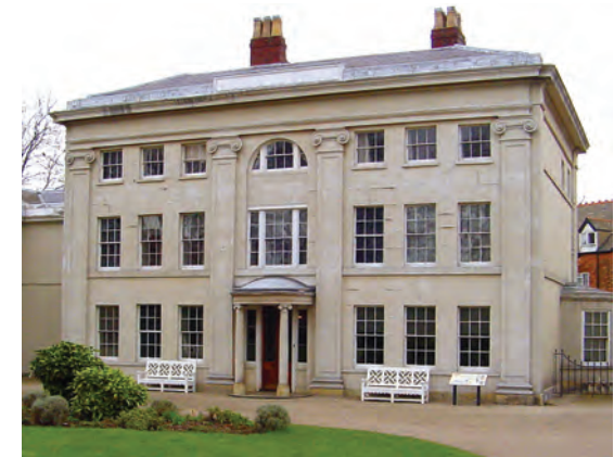
Below: Soho House, Handsworth, residence of Matthew Boulton and home of the Lunar Society.
